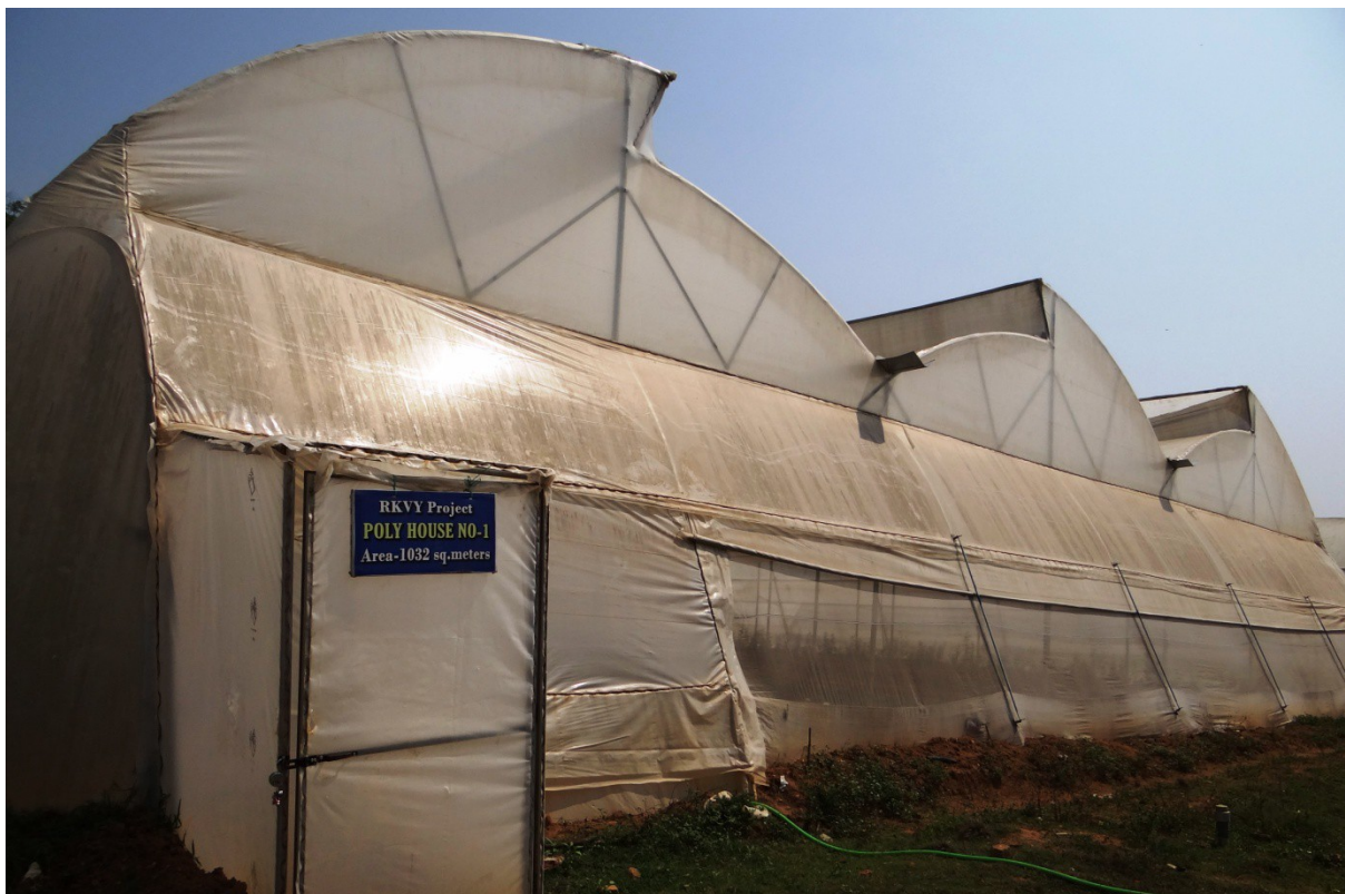
Figure 1: Naturally ventilated polyhouse erected under the RKVY project
